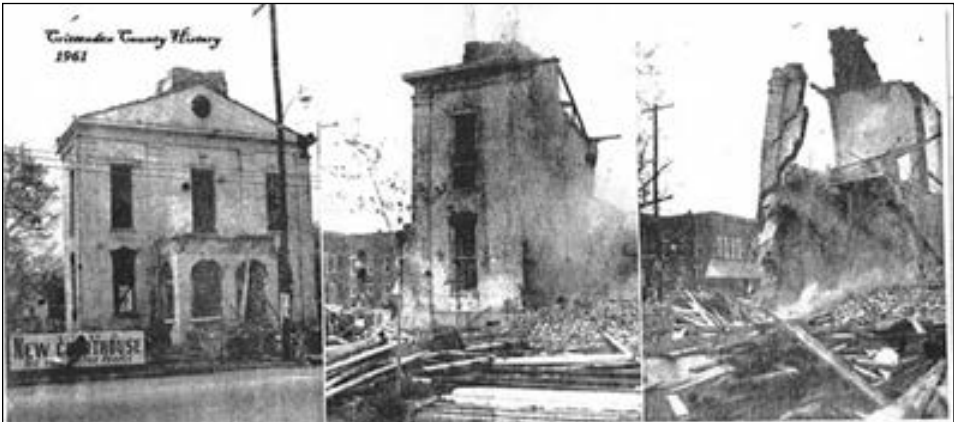
Shown are the stages of the historic courthouse as wrecker crews started tearing down its walls during the week of April 11, 1961. The walls were pulled down by a truck and cables.
